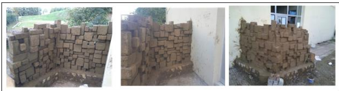
Figure 7. View of the completed wall
